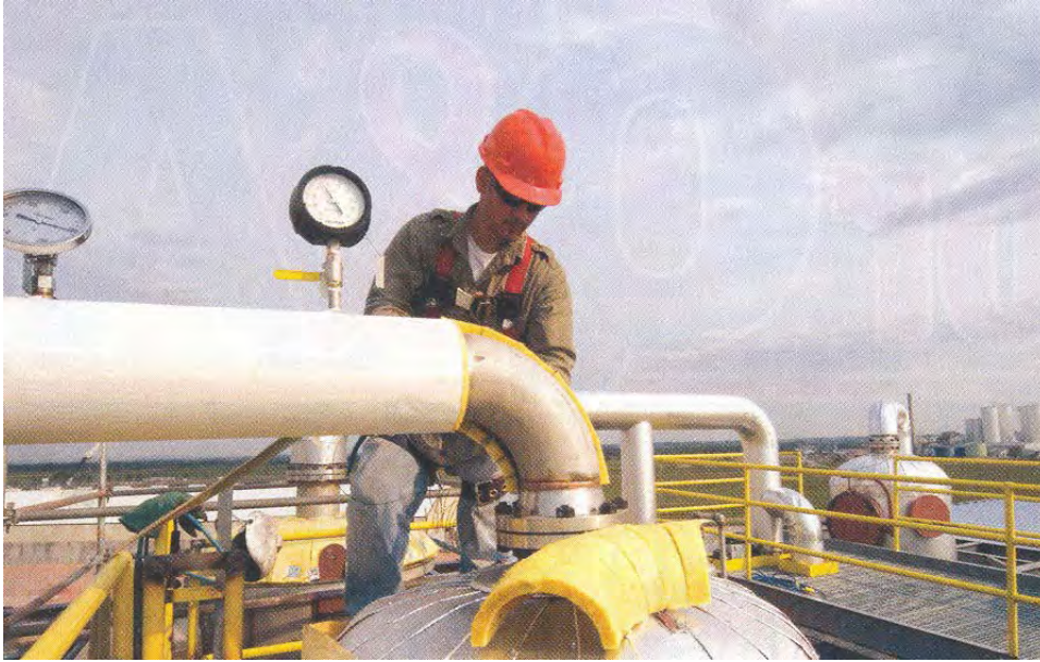
Fig. 22 Insulation of biofuel process piping
