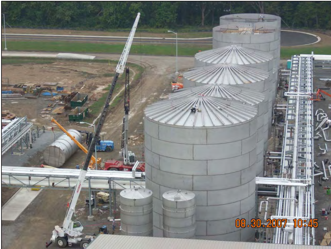
Fig. 15 View of the GO-Ethanol tanks further into construction.
